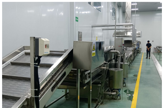
Inspection before release
